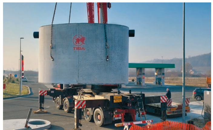
Oil separators for service stations: The gigantic containers are now also used by the Slovenian PETROL Group.
