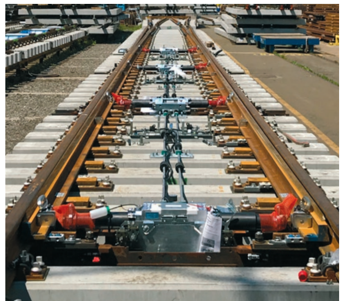
Assembly in Zeltweg: The complete set is assembled "Plug-in ready" at the production site of TSF-A joint venture partner voestalpine.
