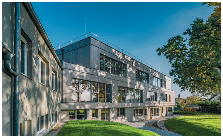
Optimal mix of materials from a single source: In Moosbrunn (Lower Austria), an elementary school building was extended using mixed precast construction. With double wall elements and element slabs, the basement was realized in concrete and the floors above in a combination of wood and precast wood-concrete composite elements.
