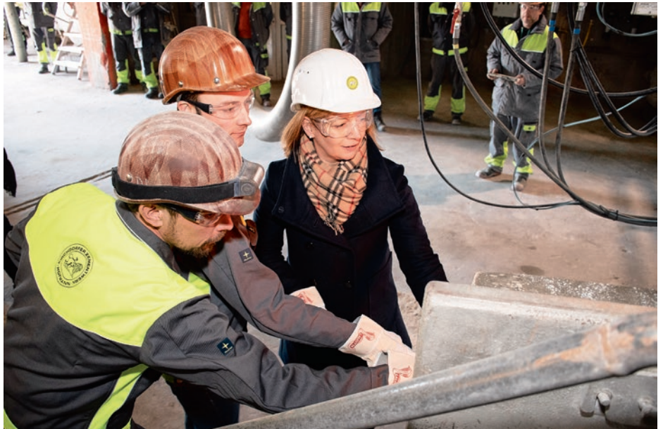
Kiln patron and district chief Elisabeth Leitner sent the Kirchdorf rotary kiln on its new journey on 10 March 2022, after the conversion work was completed. Thanks to the increased thermal efficiency of the entire system, full operating temperature was reached after only a few days this time.
