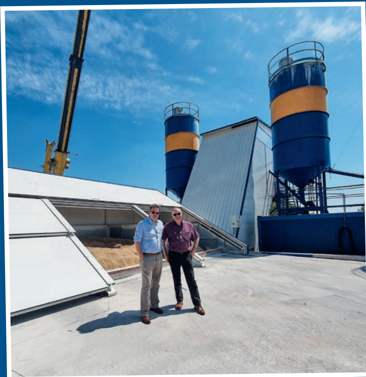
The proud managers are satisfied with the performance of the renovated plant. From left: Division Manager Armin Richter and ČRBB Managing Director Vlastimil Vrána.
